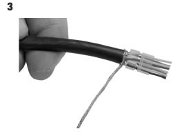
Separate all 4 pairs down to the pair spacer bar, align side by side making sure color code is correct. Insert conductors into load bar/liner.
